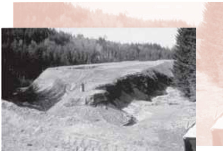
LEAD-ZINC TAILINGS DERIVED FROM A MINE IN THE SNOWDONIA NATIONAL PARK IN WALES, LAST ACTIVE IN 1954. NOTE THE SERIOUS SHEET EROSION OF THE WALLS AND THE TOP LEFT. (PHOTO: M. JOHNSON)
