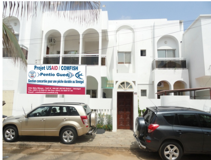
The project building with a sign consistent with the visual guidelines for the project
