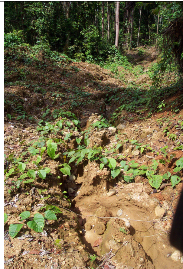
Plate 7 Erosion caused by lack of water bars.
