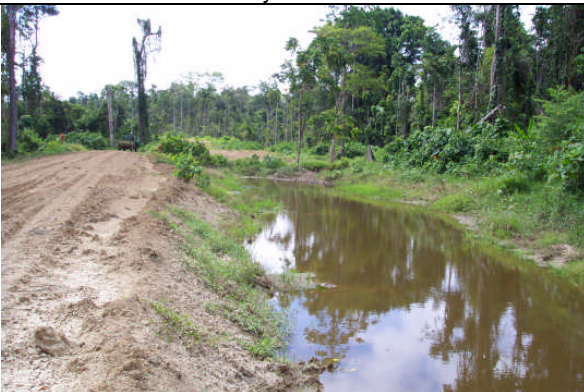
Plate 3 Lack of proper drainage causing ponding.
