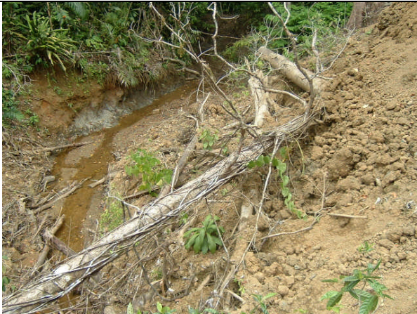
Plate 8 Excess soil and debris pushed into a Class 2 stream.
