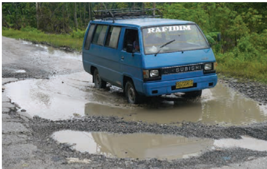
Figure 2: Potholes in tropical roads (photo © Mohammed Alamgir)
