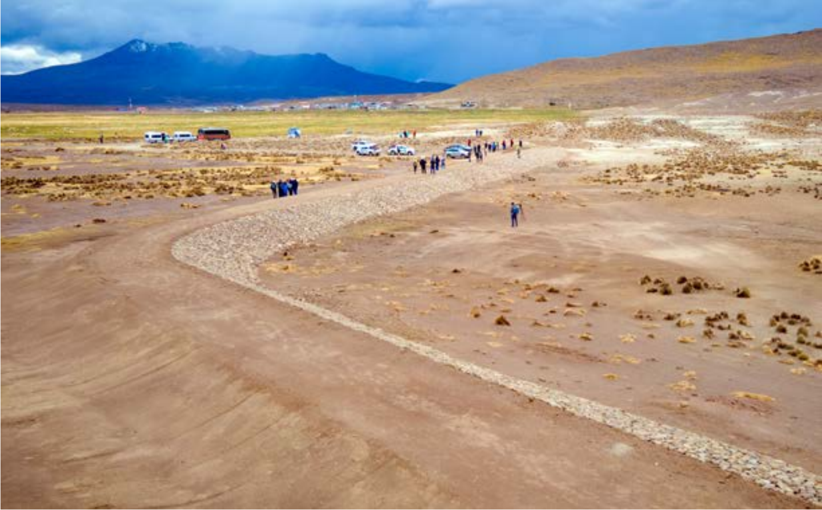
▲ Construction of permeable “micro-reservoirs,” or “qochas,” in the San Juan de Tarucani district. These qochas will collect and store water when it rains and then gradually release the water into the soil.
