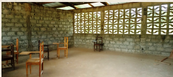
New school rooms under construction @SDI
