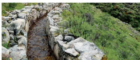
**Infiltration canals:** These transport water toward the infiltration slopes, while simultaneously allowing infiltration into the subsoil.
