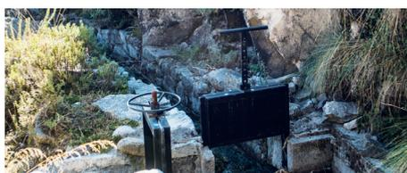
**Diversion canals:** These include two types of structures: (1) long channels that divert water flow into infiltration canals and slopes, and (2) short canals that direct the excess water towards basins or other watercourses downstream.
