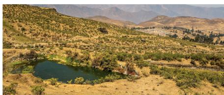
**Ponds:** Small bodies of water (around 300m<sup>3</sup> each) are used to regulate the flow of water through the infiltration system. They serve two purposes: (1) to store water for direct access, and (2) to further increase subsurface water infiltration.
