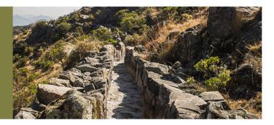
The infiltration system of the community of Huamantanga, designed to increase water available for irrigation during the dry season, and consists of the following elements:
