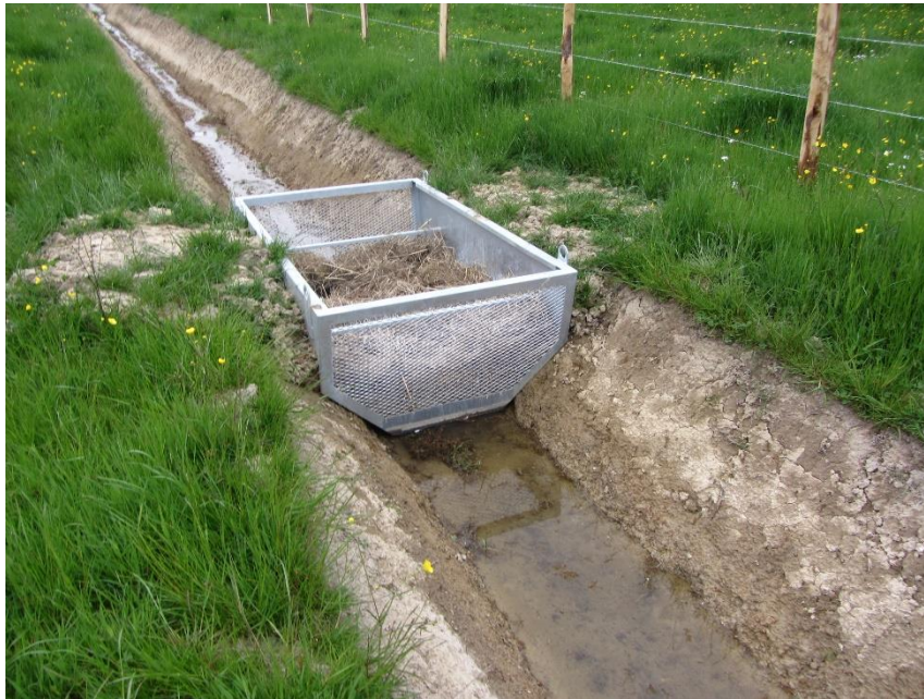
Figure 21: Temporary sanitation (Eiffage patent: Modulap®)
