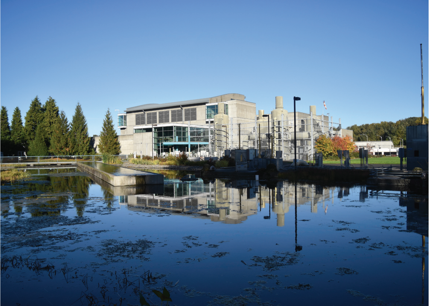
Oregon wastewater treatment plant surrounded by a constructed wetland. / Kristiana Teige Witherill
